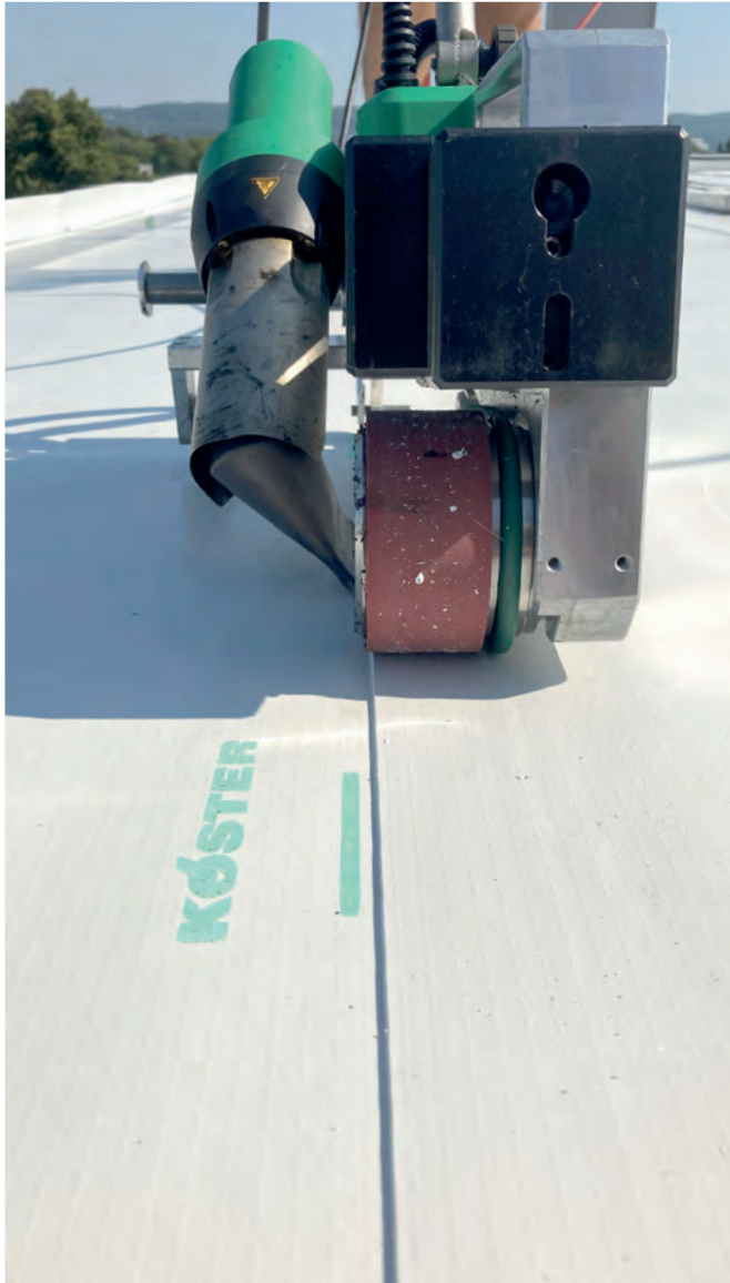
Processing by hot air welding
